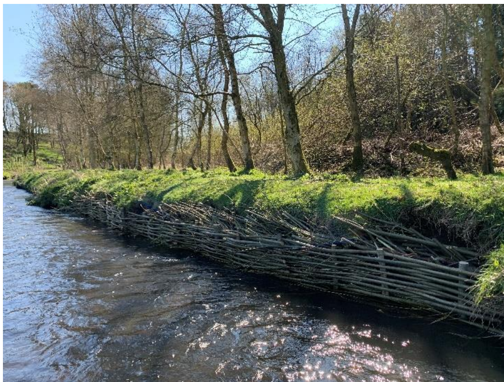
Fig 3, below showing completed Willow bank repair.
