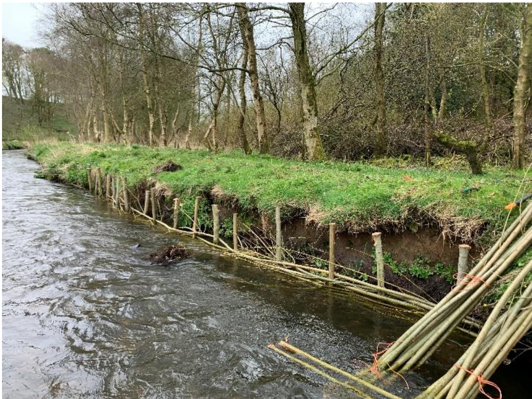
Fig 2, During bank stabilization repair below.
